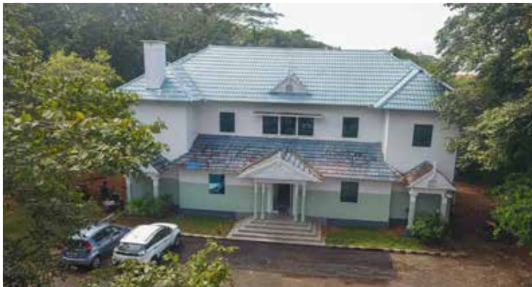
Villa IT building
